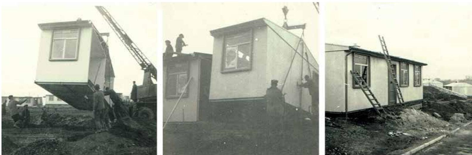
AIROH Prefab construction in Plymouth
